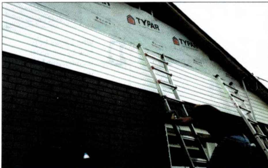
Although building paper can be used as an air barrier, it is often ineffective because of loose joints
