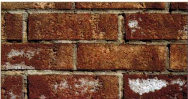
Photo 3, Efflorescence in limited areas
