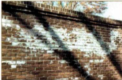
Photo 1, Efflorescence
