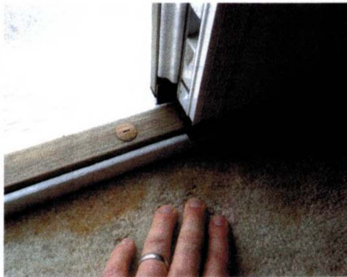
The photo above left shows a door swinging in. Water has been running down the door and wicking under the door sweep. Above right, the photo shows water-stained carpet. This house was built in 2006. This door appeared to be installed with correct threshold orientation but was still leaking — perhaps a better sweep would have kept the water out? Note the flat sill outside and wood threshold with reverse-slope — a likely problem.
