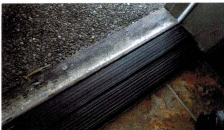
The photo above left shows a door swinging in. Water has been running down the door and wicking under the door sweep. Above right, the photo shows water-stained carpet. This house was built in 2006. This door appeared to be installed with correct threshold orientation but was still leaking — perhaps a better sweep would have kept the water out? Note the flat sill outside and wood threshold with reverse-slope — a likely problem.
