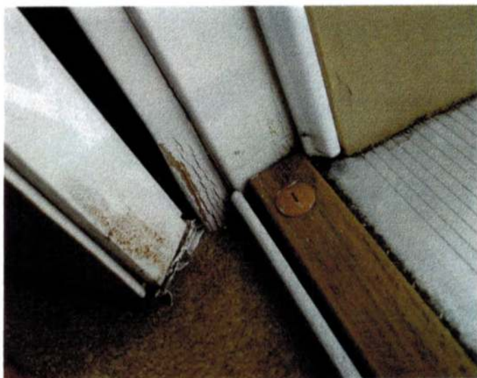
The photo above left shows a door swinging in. Water has been running down the door and wicking under the door sweep. Above right, the photo shows water-stained carpet. This house was built in 2006. This door appeared to be installed with correct threshold orientation but was still leaking — perhaps a better sweep would have kept the water out? Note the flat sill outside and wood threshold with reverse-slope — a likely problem.
