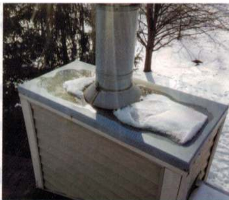
Snow, ice or water standing atop a chase cover, instead of draining, is an indicator of a poorly designed cover.
