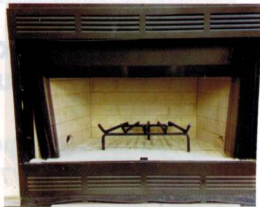
This is an example of an ideal grate size.
