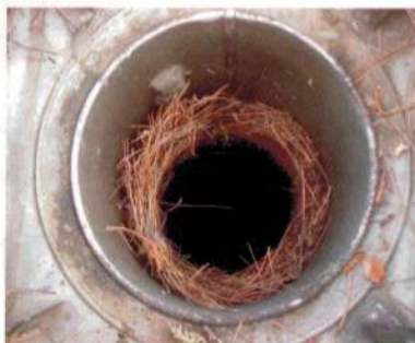
The simplest of obstructions, such as a bird's nest, can be a big issue for an unsuspecting home-owner who can't see what the home inspector can.
