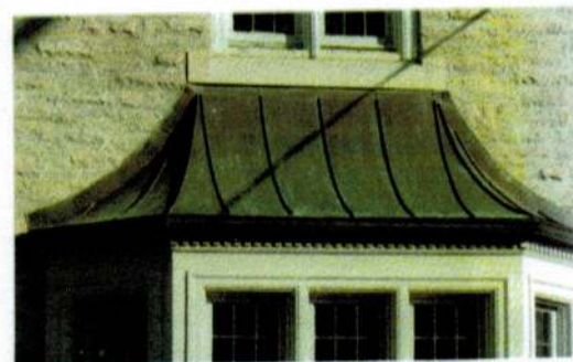
Copper roof over a bay window
