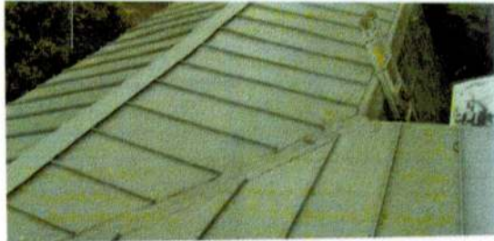
Standing seam, low-slope metal roof
