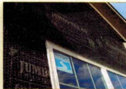
An example of proper installation of Tyvek and flashing tape around a newly installed window.
