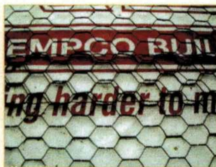
Galvanized chicken wire lath over Tyvek HomeWrap.
