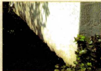
Mold growing along the rim joist due to a lack of weep screed.
