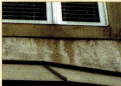
Stains at the stucco trim junctions indicate improper flashing.
