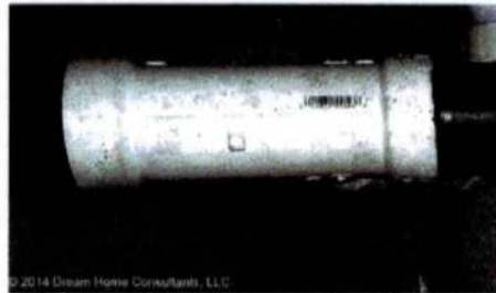
Most solvent cement connections between ABS and PVC are wrong.
