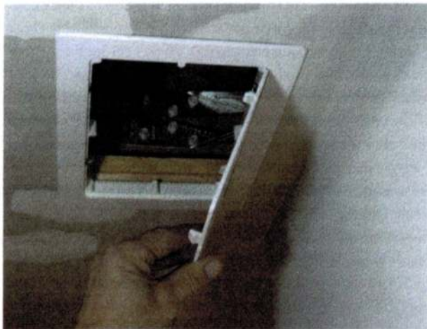
Figure 6. If you need access to install a lateral-support bracket to a house joist above a finished ceiling, using a hinged plastic panel (usually available in a supplier's plumbing department) is a quick way to cover a hole in the drywall. The panels snap into place and don't require any blocking for mounting.
