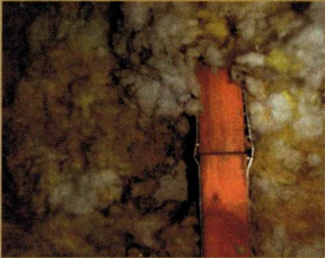
Figure 5: Compression buckling of connector plate on truss that was bent during installation (left).
