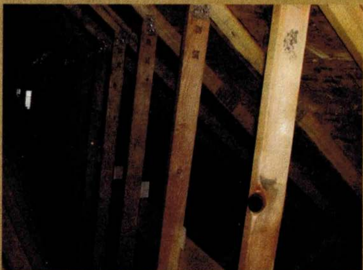
Figure 3: Knotholes weaken web members.
