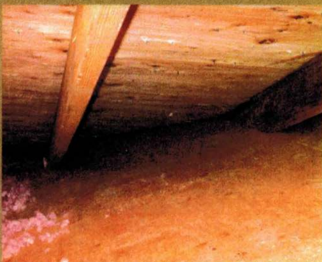
Figure 12: These rafters bear only on roof sheathing in between trusses.
