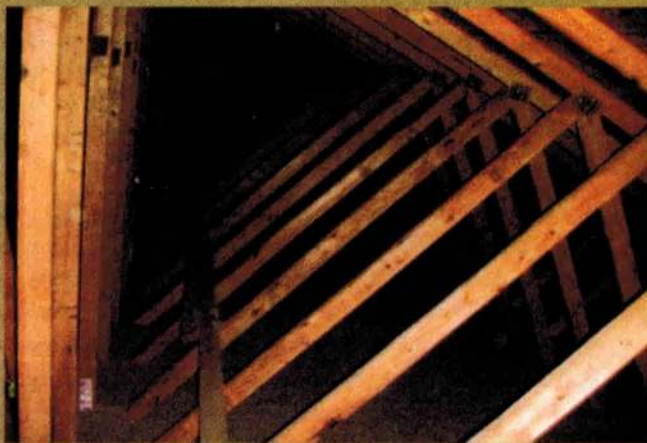
Figure 9: CLR should be roughly centered in span of web member.
