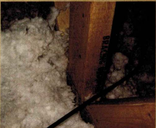
Figure 6: Ink stamp reads "BRACING REQUIRED".
