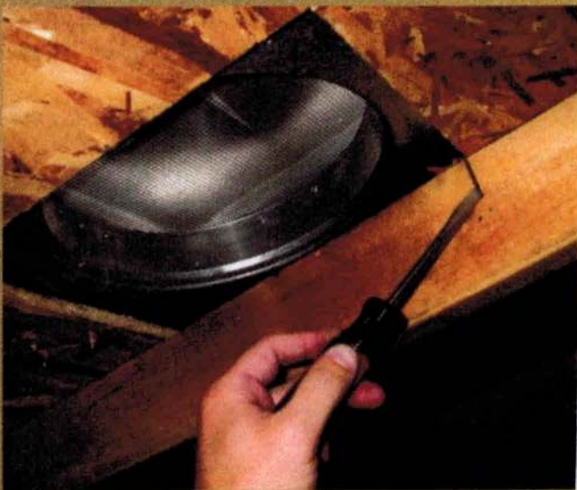
Figure 13: Truss members should not be altered in the field.
