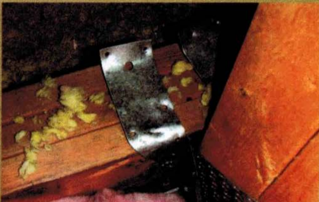
Figure 10: All nail holes should be filled in metal hanger brackets.
