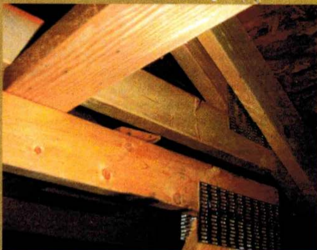
Figure 11: These piggyback trusses are not supported at the bearing point.
