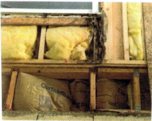
Photo 9: Sheathing is gone. (Rotted sheathing has been removed.)
