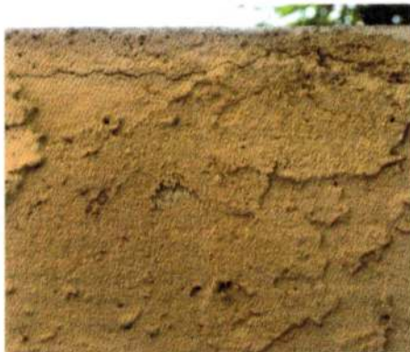
Photo 6: Here's what the home inspector can see looking up at the underside of the horizontal surface. Note the small crack and faint stains bleeding out.
