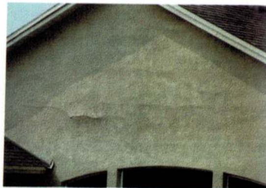
Photo 1: Parallel horizontal cracks 2 feet apart indicate improperly lapped paper-backed lath.
