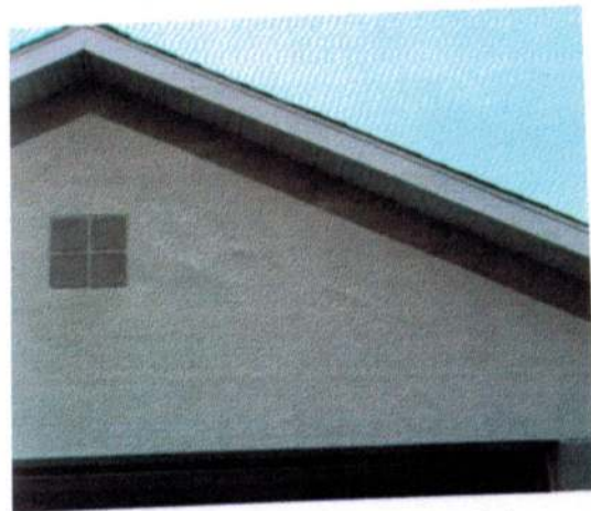
Photo 4: If you see cracking parallel to a rake edge about 2 feet down from the top of the wall, you can be reasonably sure that's due to running the lath at an angle at the top of the wall.
