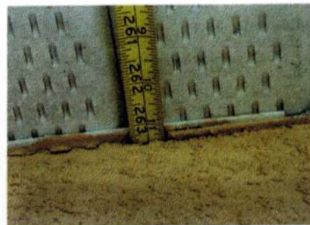
Photo 10: Measuring thickness at top of wall. Thickness here is about 5/8 inch.
