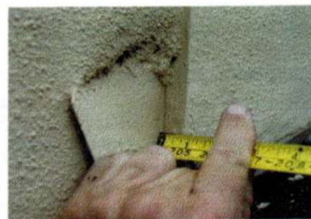
Photo 11: A 3/4-inch casing bead. The stucco cannot be 7/8 inch thick.
