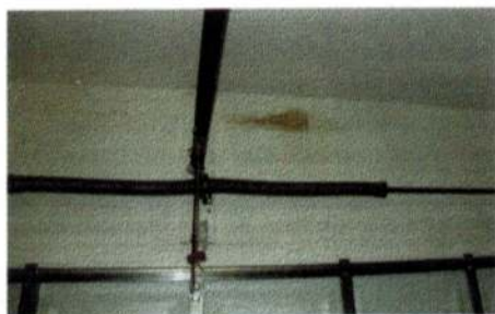
Photo 4: Water stain at the top of a garage wall below a wood frame wall. Stains like this indicate concealed damage to the wood frame wall above the masonry wall.
