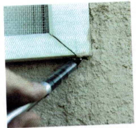
Photo 7: No casing bead and no caulked joint between window and stucco. No small cracks here. The photos that follow are all related to this window. This crack doesn't look like much, but the resulting damage is impressive.
