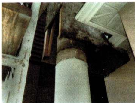
Photo 7: Here's what the structure looked like after the stucco was removed. If you can see stains bleeding out, it's very likely there's heavy damage.
