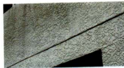
Photo 3: No weep screed at bottom of second story wood frame wall. Casing beads do not drain water.
