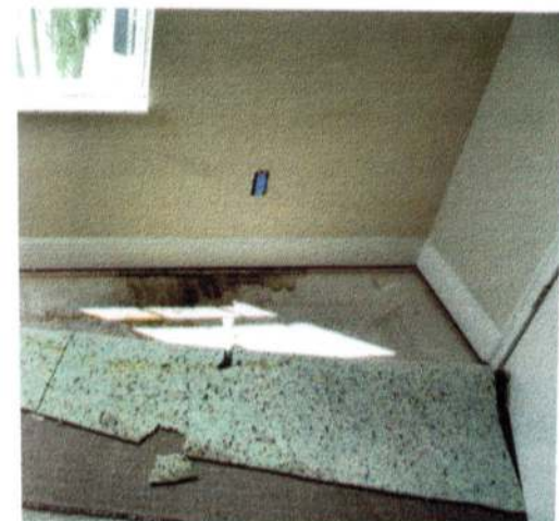
Photo 11: I always pull up the edge of carpeting below windows using needle-nose pliers. If I see staining, I know there's concealed damage in the walls. In this case, I was inspecting stucco for the owner and was able to pull back the carpeting, revealing the large stain on the floor.
