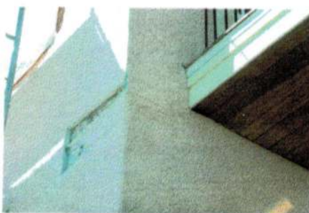
Photo 13: It's not just windows; all dissimilar materials intersecting stucco need casing beads and caulked joints. This intersection of a fascia and the stucco wall didn't show any signs of damage other than some staining on the wood ceiling.
