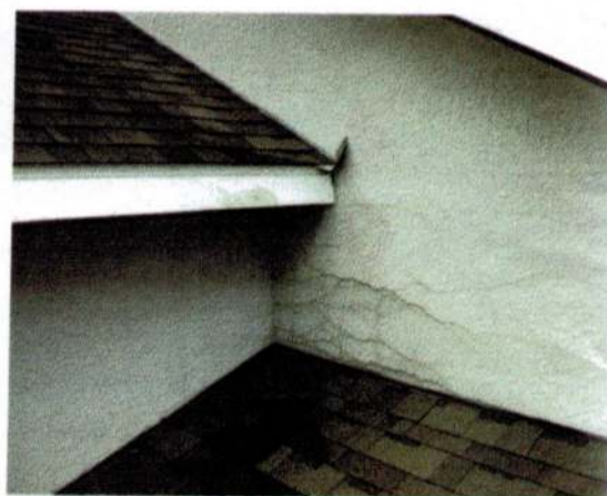
Photo 16: This cracking is caused by multiple issues: water entry at the kickout flashing that's not caulked, stucco that's too thin and improperly lapped paper-backed lath.
