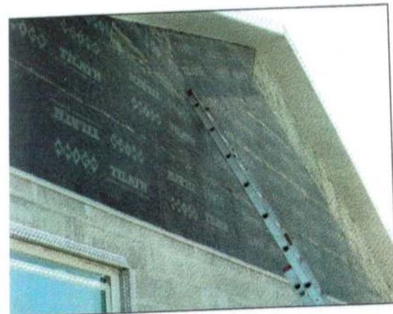
Photo 5: Lath run at an angle overlapping the horizontal pieces causes cracking at the thin areas created by improper lapping.
