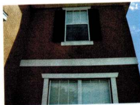
Photo 1: No drainage at bottom of second story wood frame walls above first floor masonry walls.
