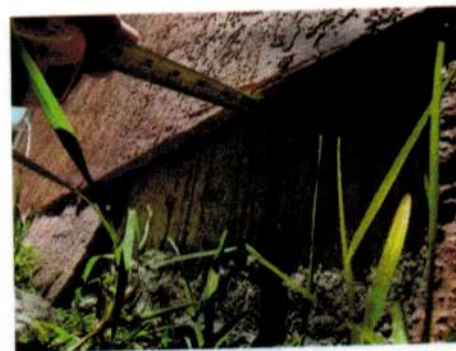
Photo 2: No weep screed at bottom of first floor wood frame wall. Casing beads do not drain water.
