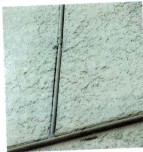
Photo 6: Separation at control joint. The crack here admits water, which causes lath to rust and expand, leading to more cracking and damage.
