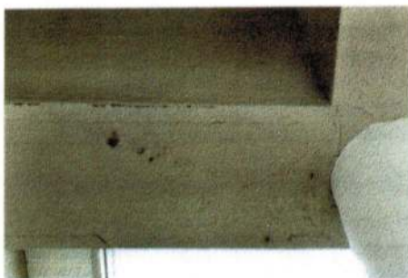
Photo 8: If you see this on the underside of a horizontal return, you can be certain there's heavy damage.
