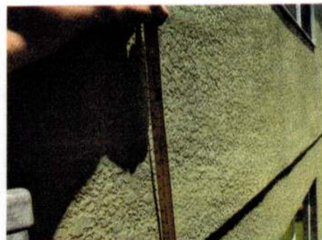
Photo 12: Stucco gets noticeably thinner away from accessories such as weep screeds and control joints.
