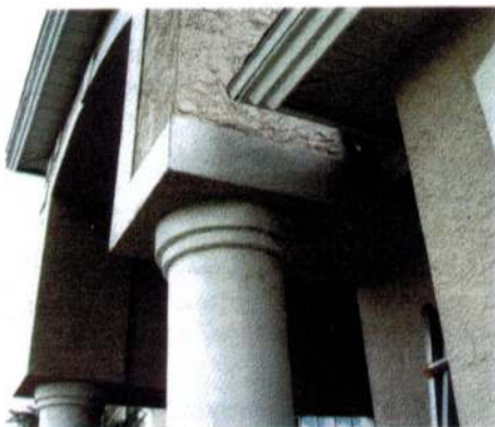
Photo 5: No drainage at horizontal return below vertical stucco walls.
