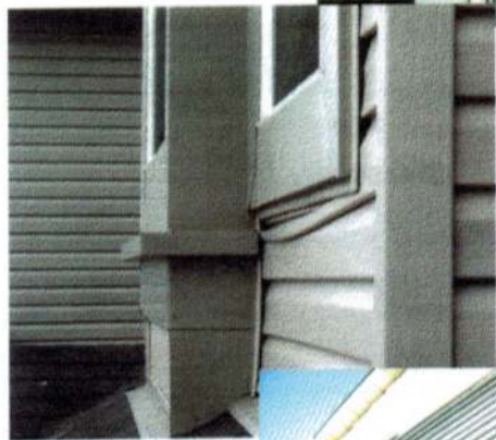
Siding is poorly secured.
