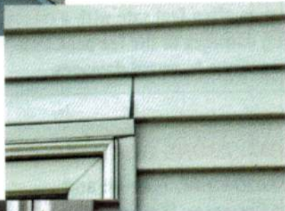
Siding is not well secured below window.
