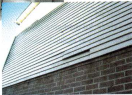
Siding is poorly secured.
