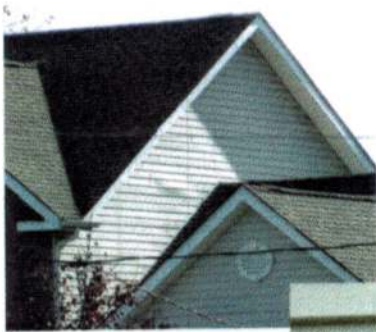
Siding in danger of blowing off; pieces are not interlocked properly.
