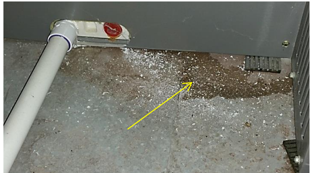
Leaking condensate tray
