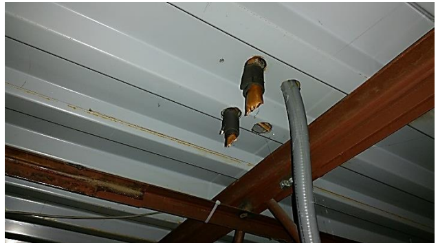
Disconnected refrigerant pipes
