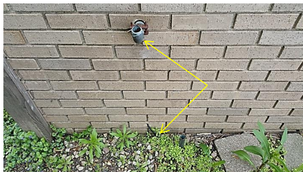
Disconnected sprinkler
