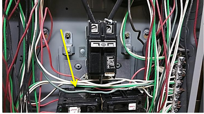
Wires crossing bus bar
