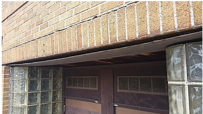
Rusted & sagged steel lintel
