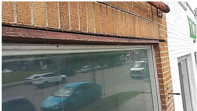
Rusted & lifted steel lintel
