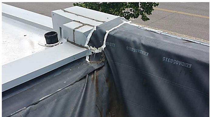
Loose, wrinkled, & caulked membrane
