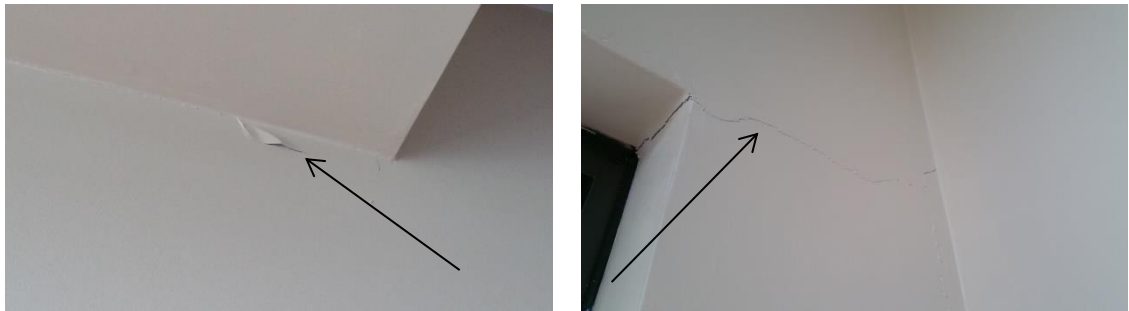
Cracked plaster / torn paper tape
