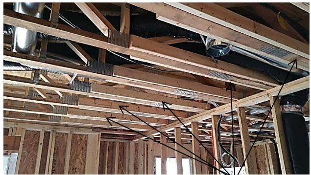
Broken trusses
