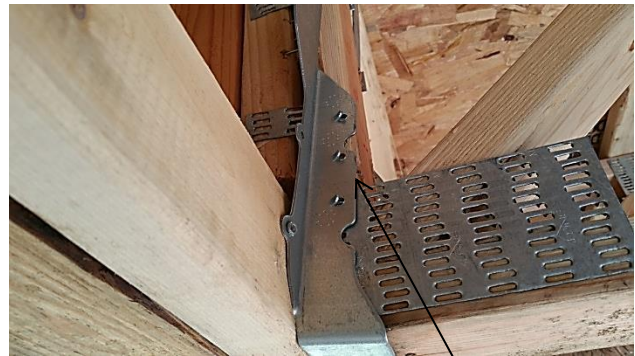
Joist hanger nails
