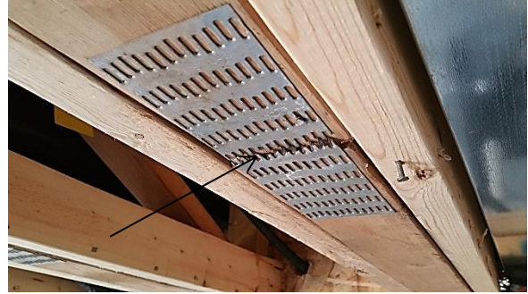
Damaged gusset plates
