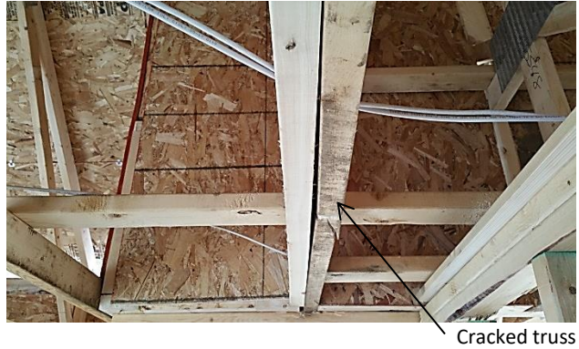
Cracked truss
