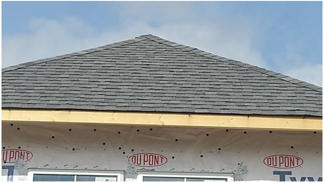
Buckled, lifted, & uneven shingles
