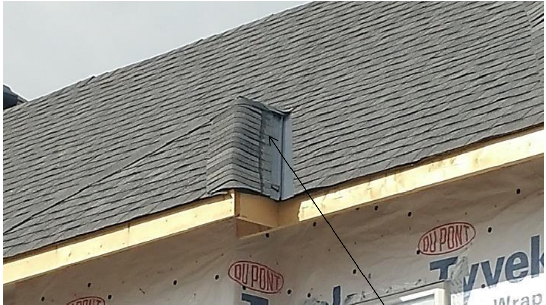
Poorly installed valley shingles
