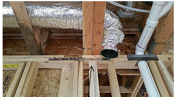
Main level beam end bearing
