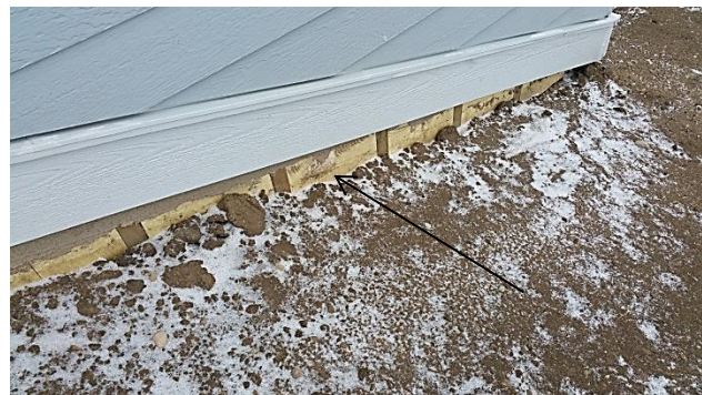
Exposed styrofoam
