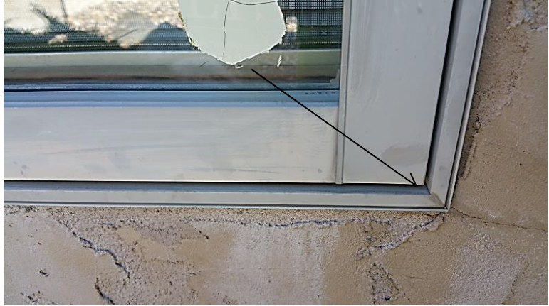
No corner joint caulking
