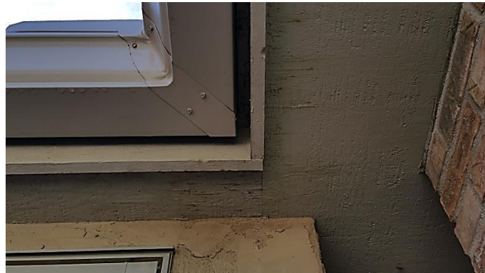
Water damaged soffit (front)
