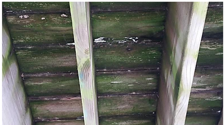
Decayed floor boards
