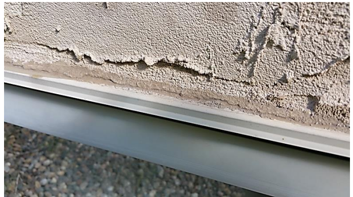
Caulked window top (traps moisture)
