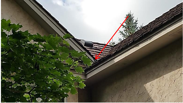
Restricted drainage (ice dam)
