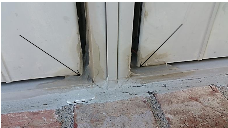
Excessive corner caulking (front only)
