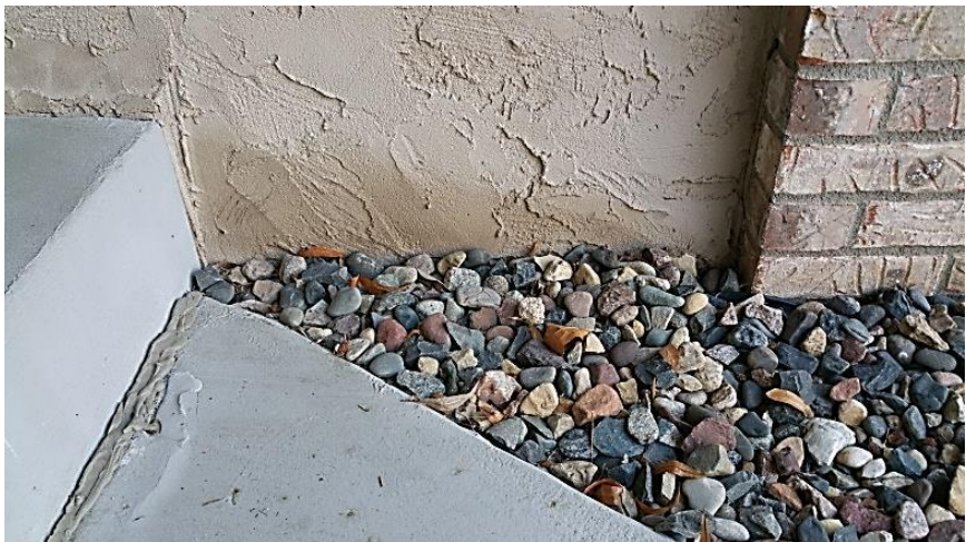
Stucco contacting earth
