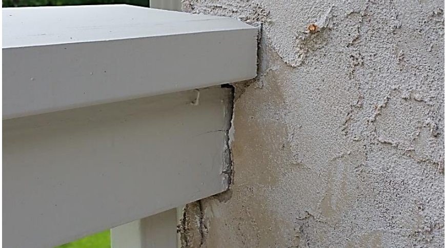
Guardrail in stucco (moisture intrusion)
