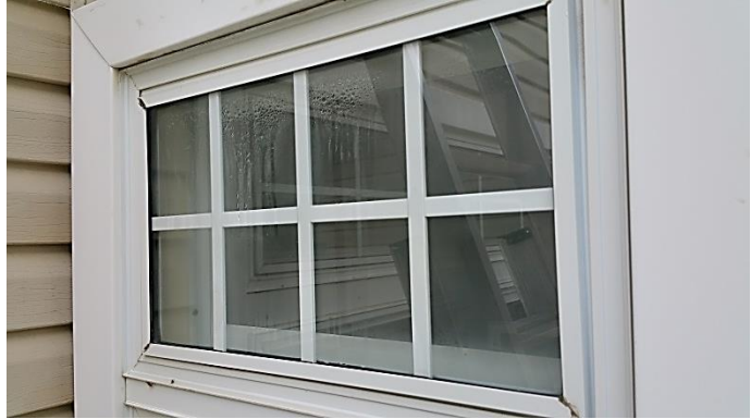
Leaking glass
